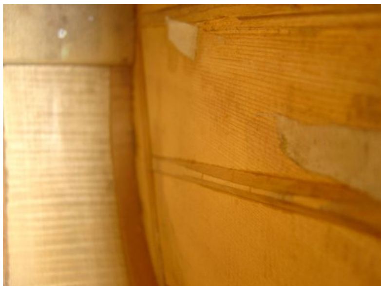
Figure A 19. Interior view of the center fan brace and one bass fan brace (photo courtesy James Westbrook)
