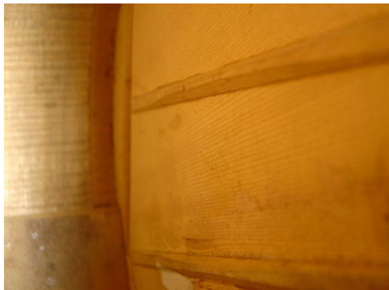
Figure A 18. Interior view of the center fan brace and one treble fan brace (photo courtesy James Westbrook)
