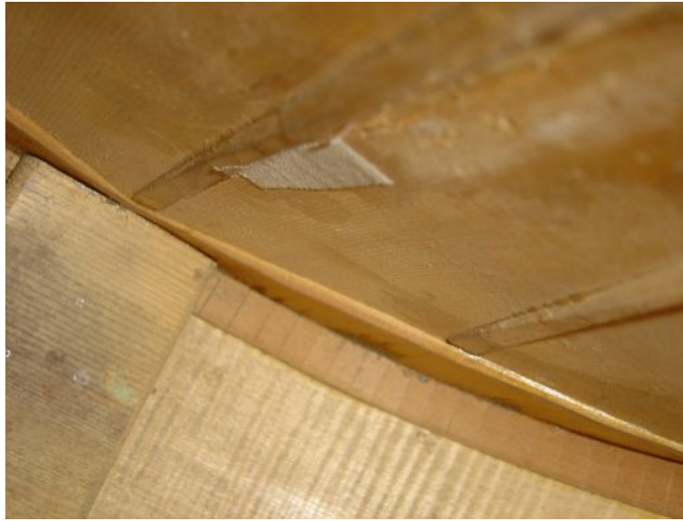
Figure A 21. Interior view of the center fan brace, cloth patch and tail block, focus on the tailblock (photo courtesy James Westbrook)
