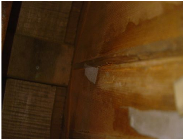
Figure A 22. Interior view of damage on the top and center fan brace (photo courtesy James Westbrook)
